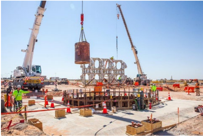
A bucket of excavated dirt is lifted out of the utility shaft being excavated at WIPP.
