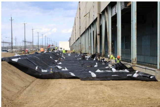
Workers install liner in the water retention berm as an infrastructure support and safety measure during X-326 Process Building demolition.
