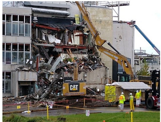
A heavy equipment operator removes and size-reduces concrete and steel during the demolition of the Main Plant Office Building. In the foreground, workers prepare to remove a full waste container from the demolition area.
