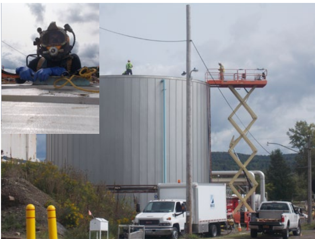
Professional divers enter the top of West Valley's 40-foot Fire Water Storage Tank to perform underwater inspections, cleaning, and repairs.
