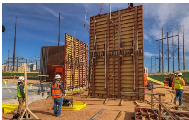
As part of the SSCVS, concrete forms are installed in preparation for construction of the Salt Reduction Building.
