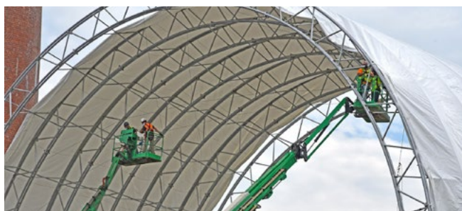
Crews installed a six-story protective cover over the final hot cells remaining from Building 2026 in the central campus area of ORNL. This cover will allow EM to demolish the structures while ensuring no impact to the nearby research and science missions.
