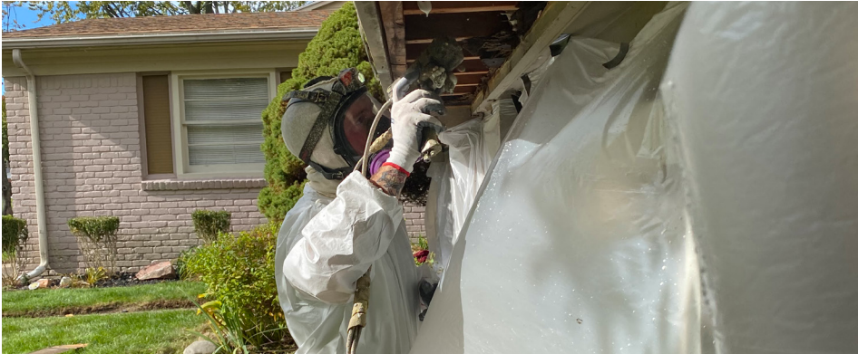
An installer with Ecotelligent Homes installs spray foam around the perimeter of the upper level, which cantilevers over the lower level.
