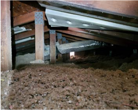
The upper attic was air sealed and insulated to R-49. New six-foot baffles facilitate attic ventilation.
