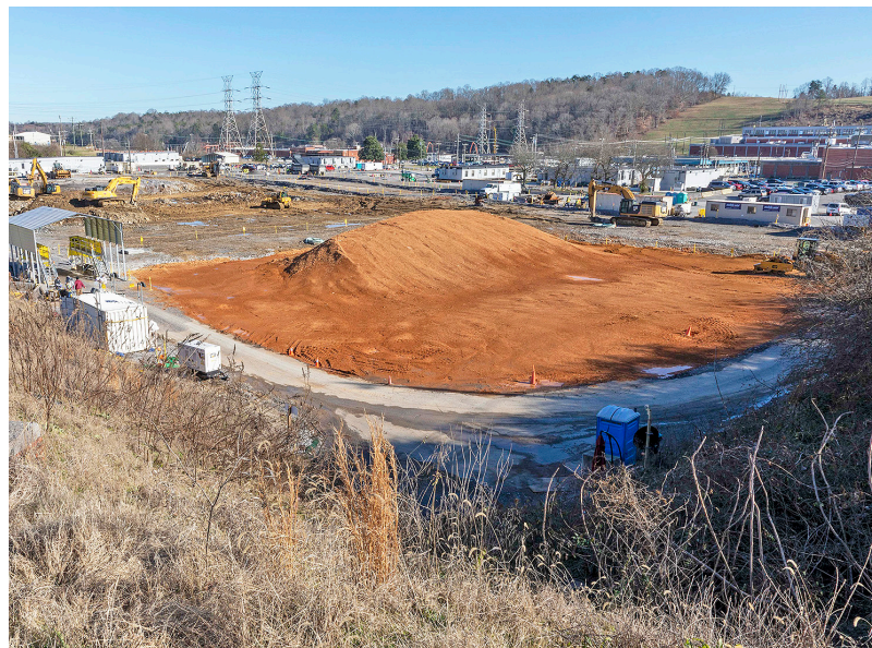
Soil is brought in to backfill the former Biology Complex area after slab removal.
