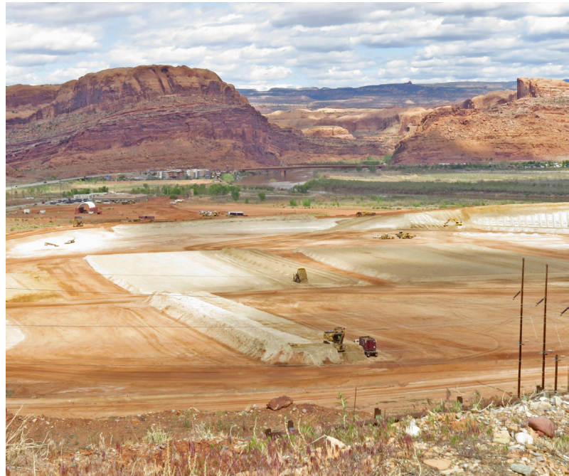
The Moab site tailings “pile.” Rows of tailings are dried out before being loaded into specialty train containers, which are carried by haul trucks to the train and then loaded and transported to the disposal cell.
