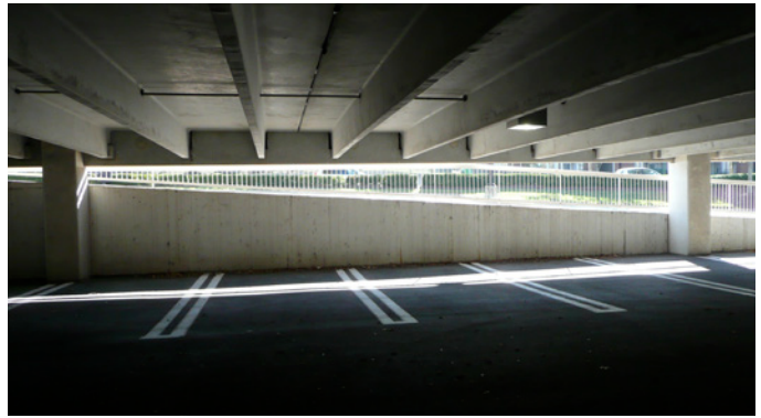
Figure 8(d). Photo – typical ceiling construction
