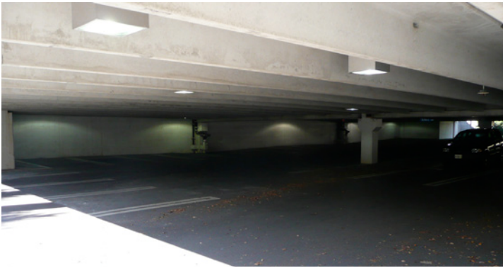
Figure 8(b). Photo – entrance during the day
