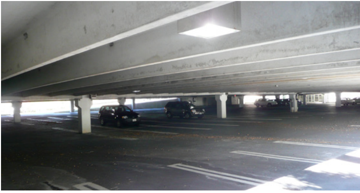
Figure 8(a). Photo – perspective of the parking structure
