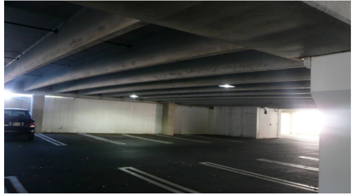
Figure 8(c). Photo – corner of parking structure
