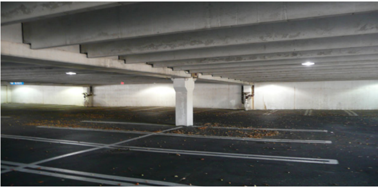
Figure 9(a). Photo of site
